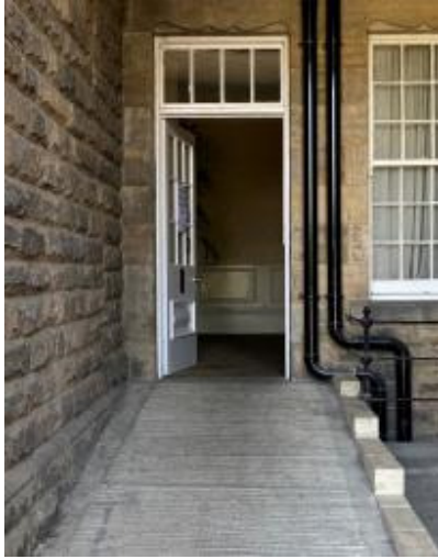
Outside ramp entrance to fitness room & meeting rooms
