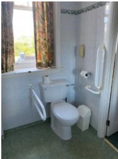
Toilet in room 137
